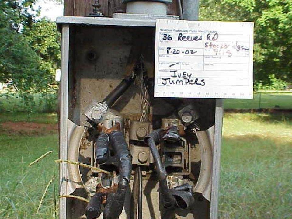
Auto jumper cables being used to jump out service.
