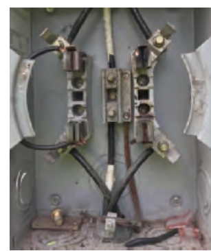
Figure 4: Remnants of a load-to-load short and socket damage discovered at a single-family home.
